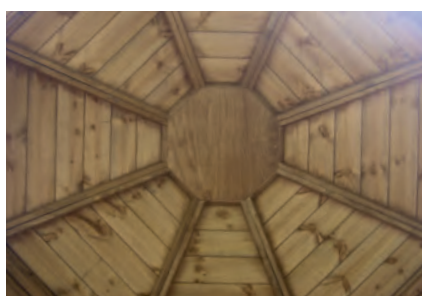
Internal roof structure
