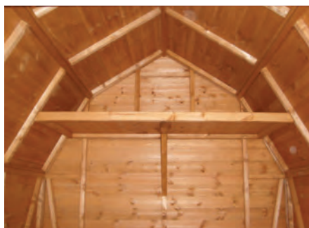
Internal roof and shelf
